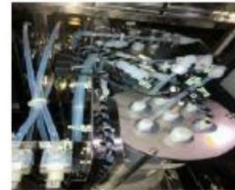
HMDS Buffer Tank
